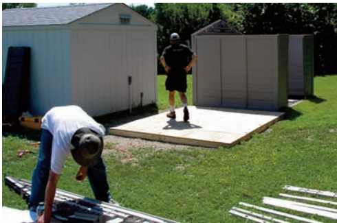
New storage shed, July 2008
