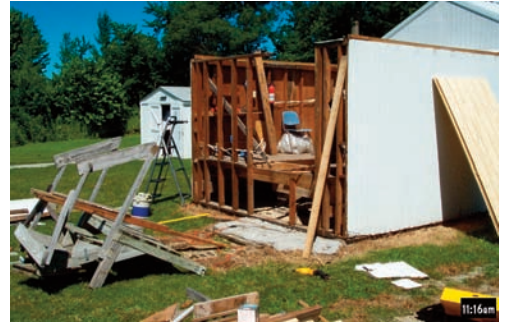
Observatory siding replacement and wall repair - July 2008
