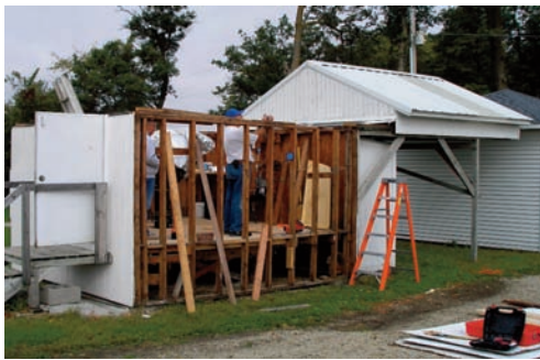
East side of observatory repaired Sept 2010
